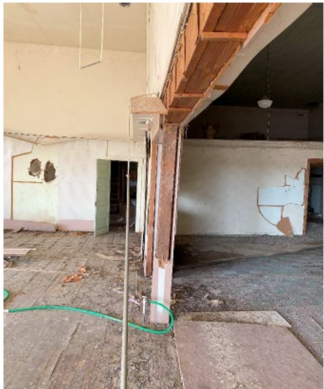
LOCATION OF WORST FLOOR SETTLING AND DISPLACED ROOF SUPPORT
