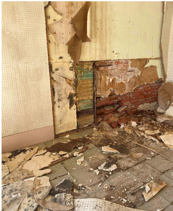
INTERIOR DELAMINATION AND FALLING BRICK WITH DETERIORATED MORTAR
