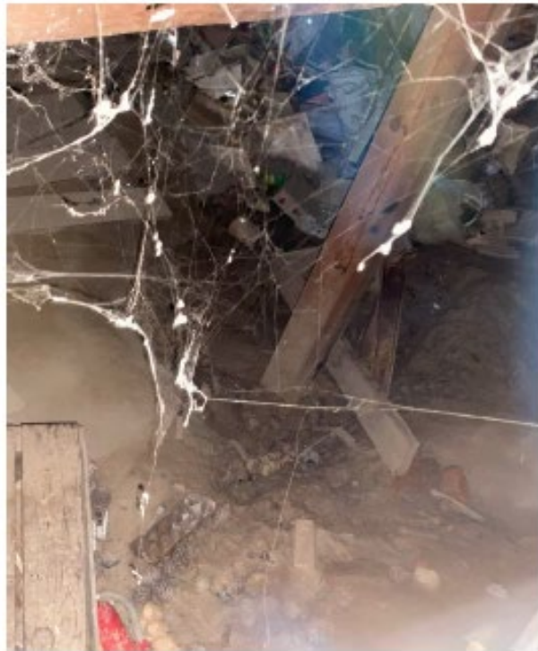
CONDITION OF FLOOR FRAMING AND SUB-FLOOR POST WITH SETTLEMENT (Requires Modification/ Repair)
