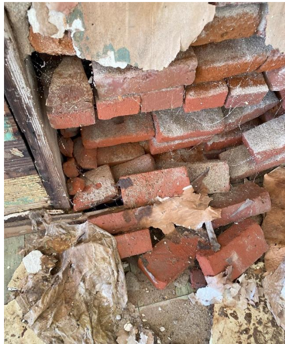
INTERIOR DELAMINATION AND FALLING BRICK WITH DETERIORATED MORTAR
