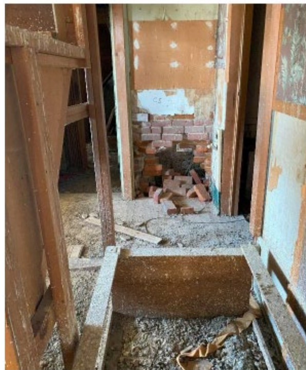
ADDITIONAL MORTAR DEFICIENCY AND BRICK DELAMINATION
