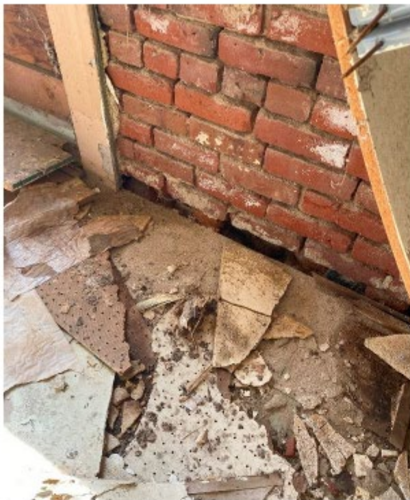
ADDITIONAL MORTAR DEFICIENCY AND BRICK DELAMINATION
