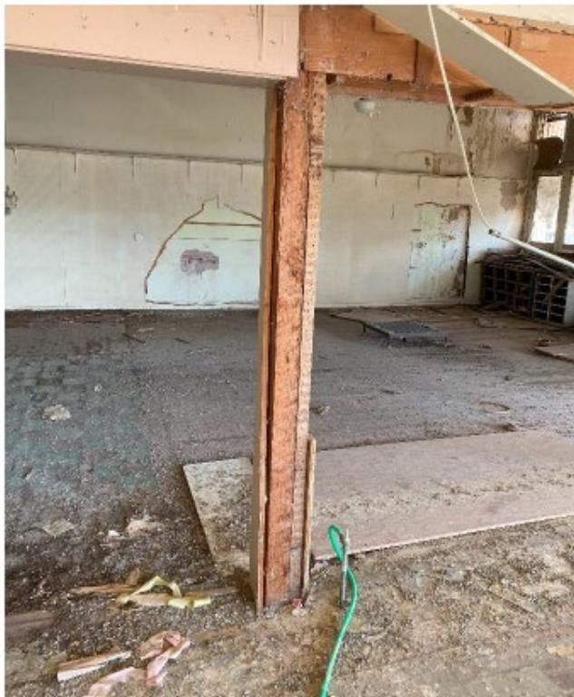
LOCATION OF WORST FLOOR SETTLING AND DISPLACED ROOF SUPPORT
