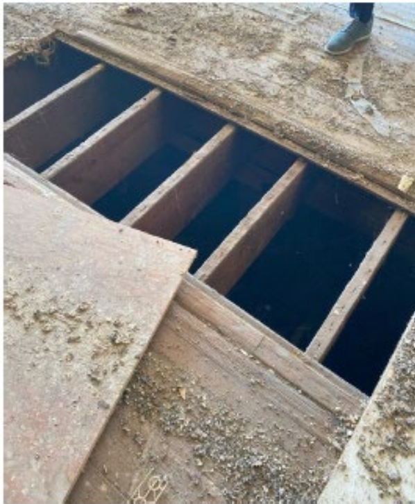
CONDITION OF FLOOR FRAMING AND SUB-FLOOR POST WITH SETTLEMENT (Requires Modification/ Repair)
