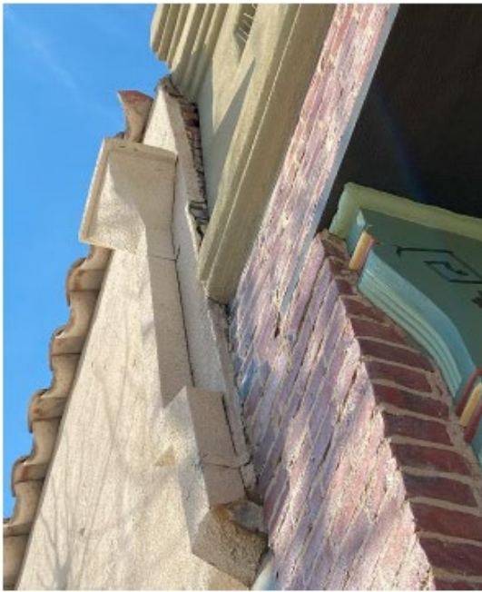
LATERAL DISPLACEMENT OF BUILDING PARAPET AT CORNER AND EXPOSED BRICK
