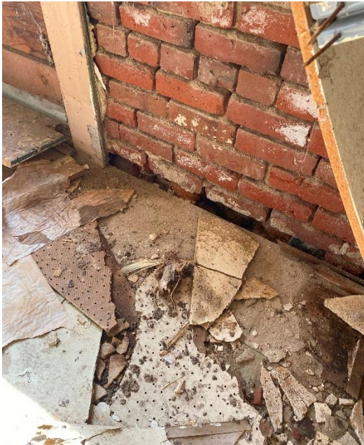
ADDITIONAL MORTAR DEFICIENCY AND BRICK DELAMINATION
