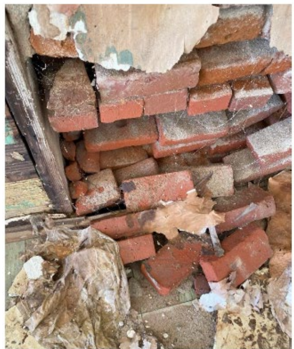
INTERIOR DELAMINATION AND FALLING BRICK WITH DETERIORATED MORTAR
