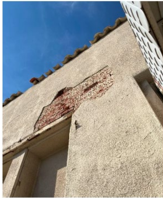
LATERAL DISPLACEMENT OF BUILDING PARAPET AT CORNER AND EXPOSED BRICK
