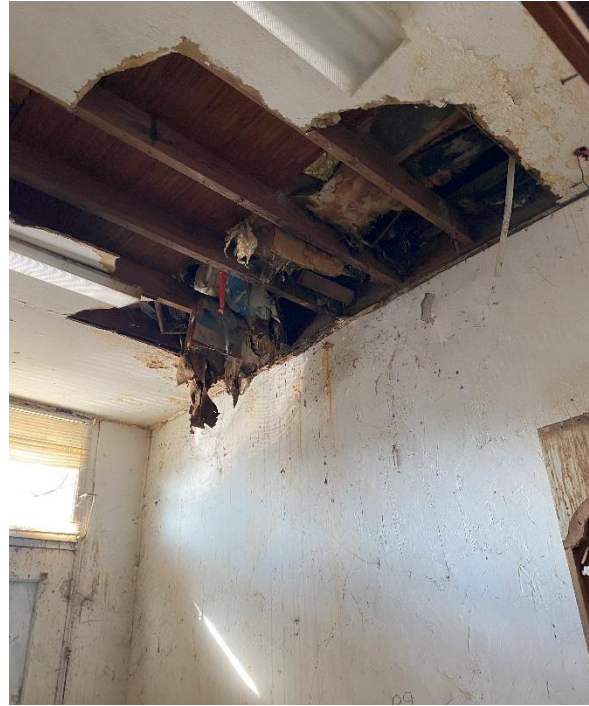
CONDITION OF VISIBLE ROOF FRAMING
