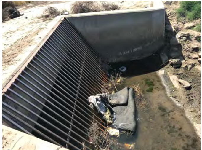
View of existing Peoples Ditch culvert inlet that goes underneath Highway 198, facing south. Visible signs of debris and human disturbance were observed within the canal. April 27, 2020.
