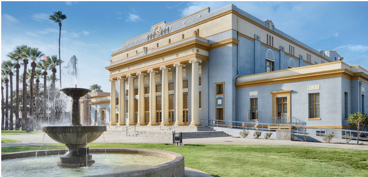
Figure 2: Civic Auditorium: 400 N. Douty Street
