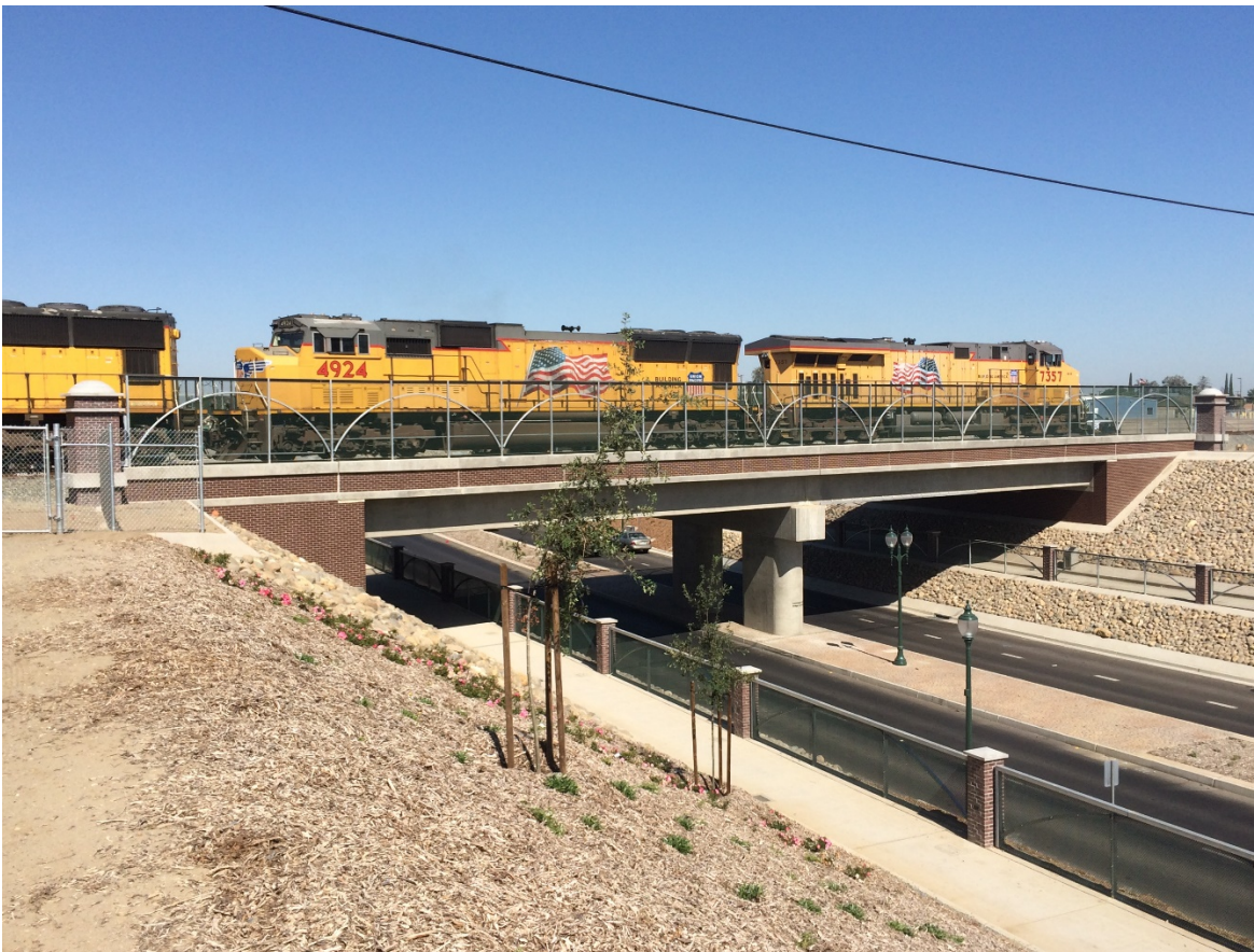
Figure 3: Underpass Structure; with retaining walls (above), with cut slope (below)
