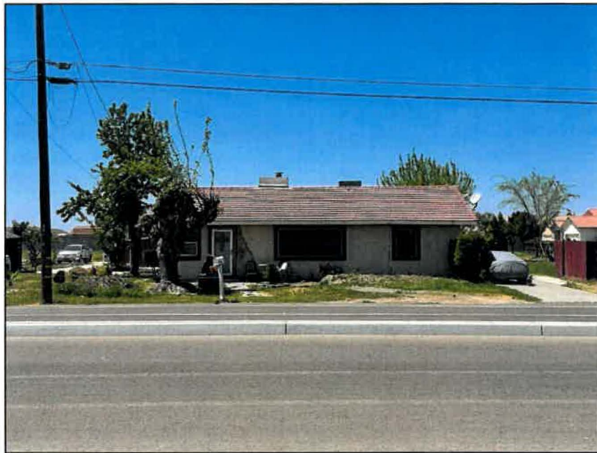
View of the single-family residence and front yard looking west across the 12 th Avenue frontage.
