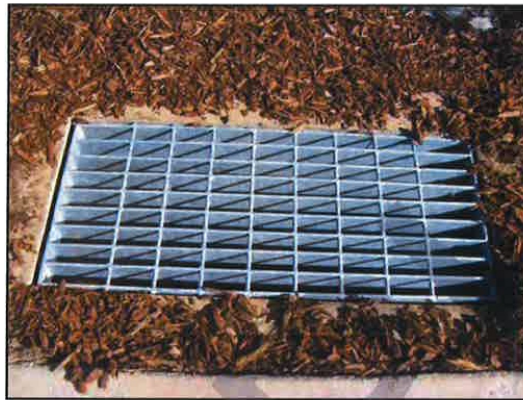
Storm Drain Inlet
