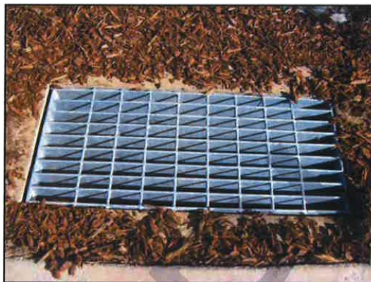
Storm Drain Inlet
