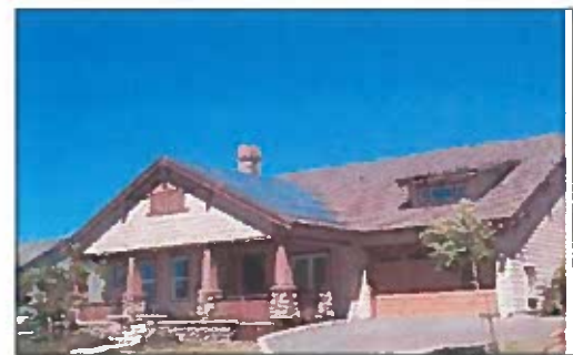
An example of PV Panels on a residential unit
