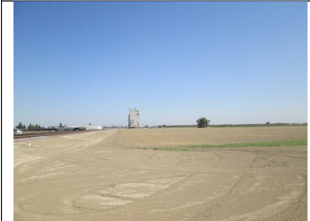
North view of rail road
