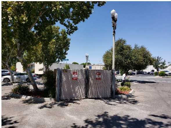
Trash enclosure and lighting
