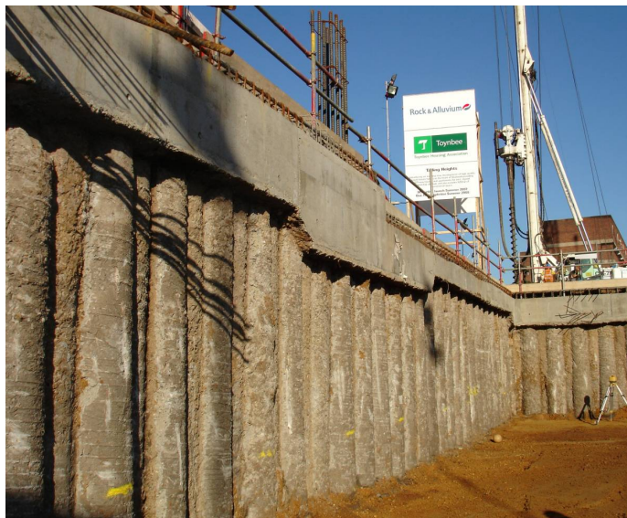
Figure 7: Example Secant Pile Wall without Fascia
