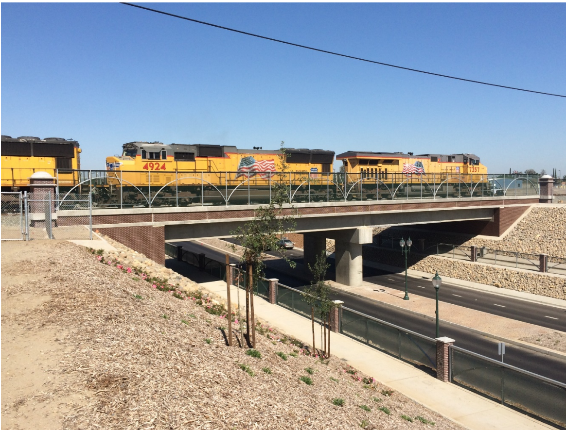
Figure 3: Underpass Structure; with retaining walls (above), with cut slope (below)
