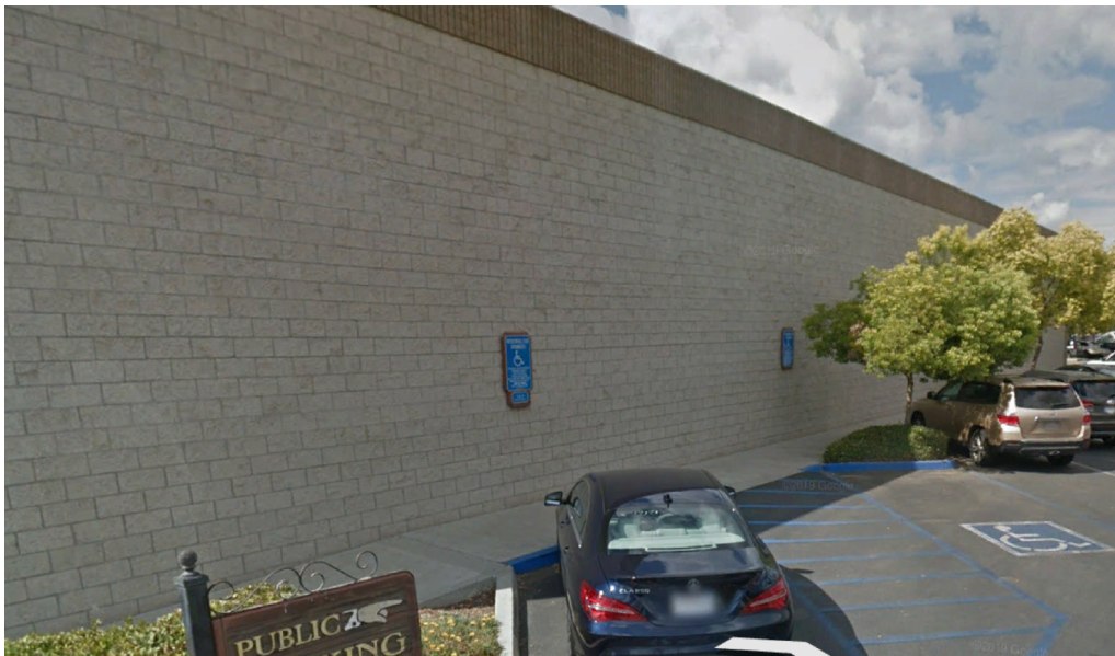
PARKING LOT / CITY OF HANFORD'S CMU WALL
