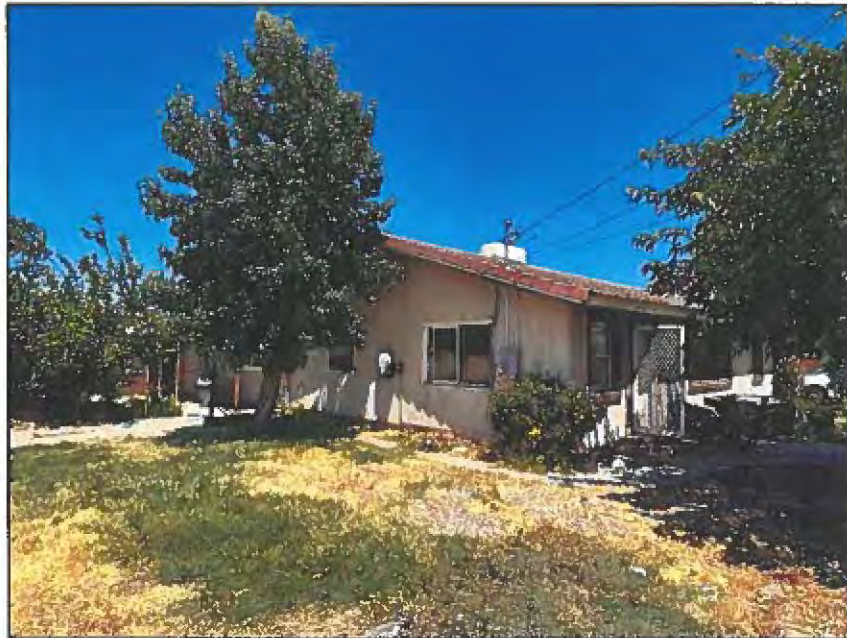
View of the house showing the front and south side elevations.
