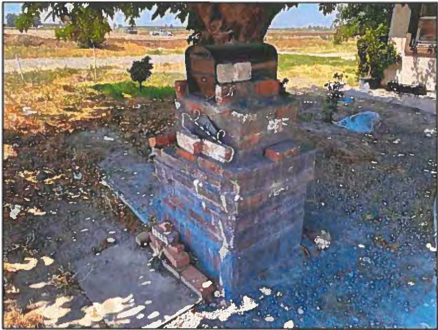
View of the mailbox on a brick base that is located in the ROW take area.
