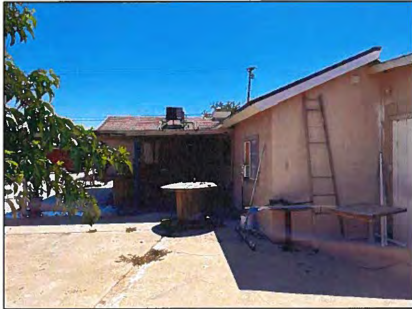
Rear view of the house and the attached carport.
