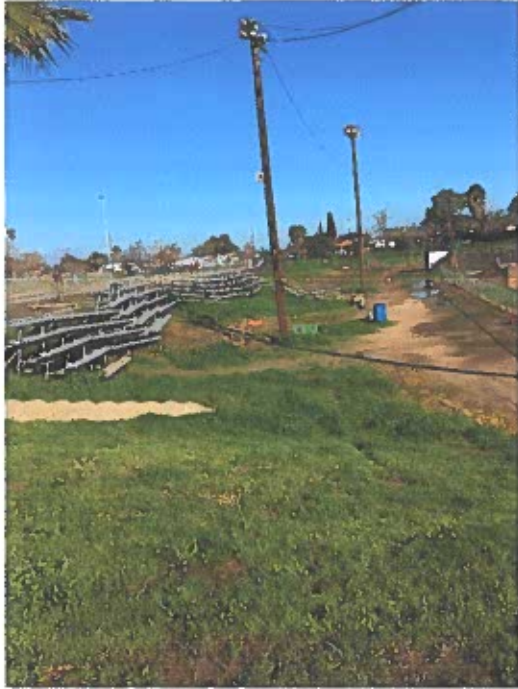
Overgrown grass and broken bleachers when we took over track
