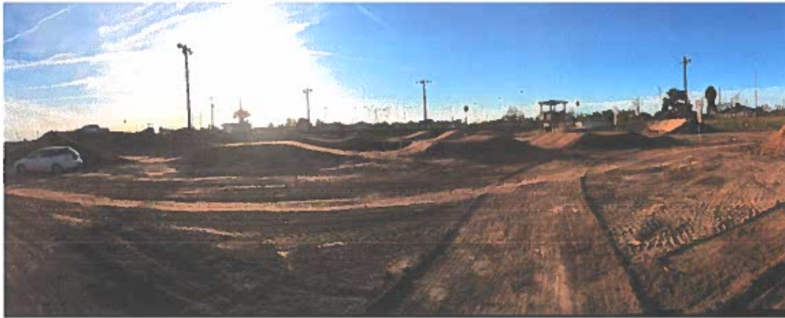
Below: Track rebuild, and building strider track
