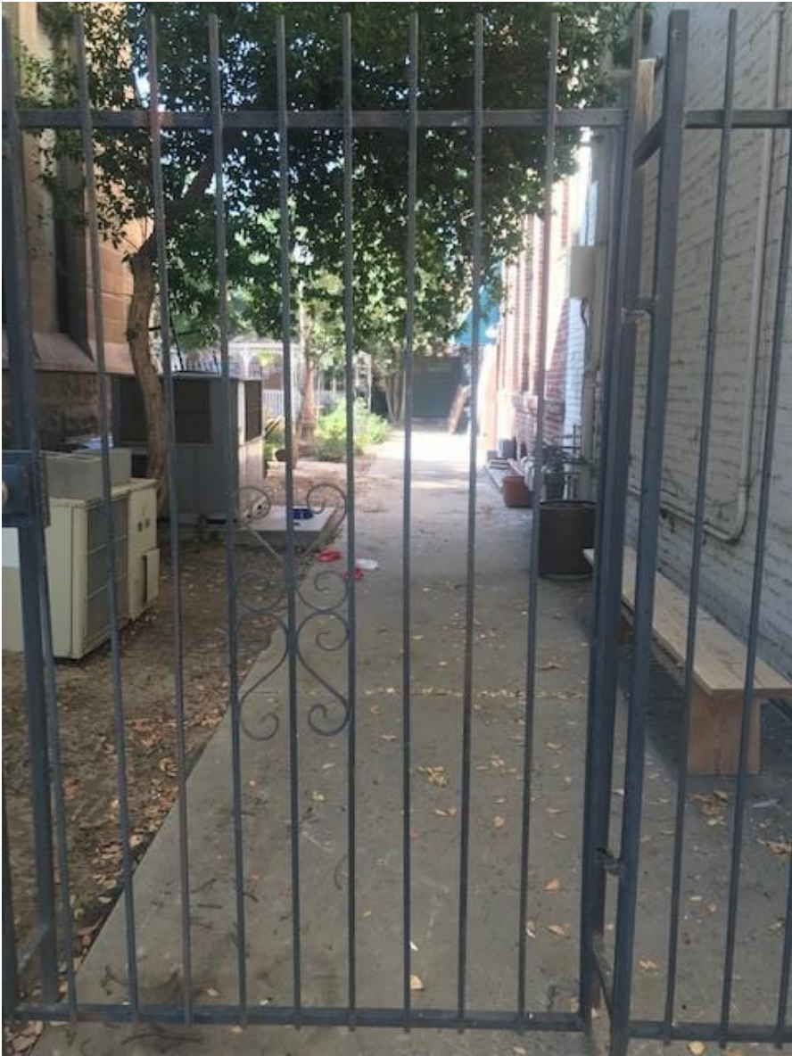
Photo of west side of building
