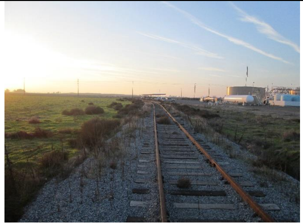
Northern parcel rail spur
