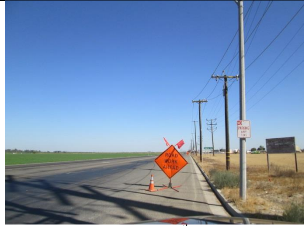
North view on 11 th Avenue
