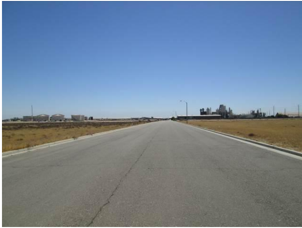
Looking east along Energy Street
