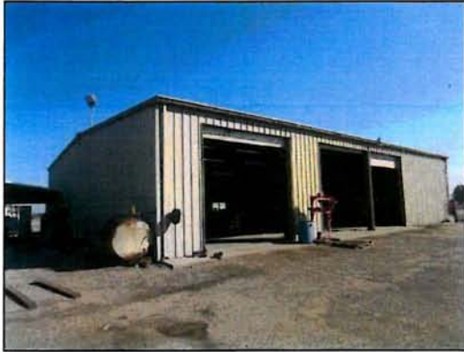
View of the repair shop building.
