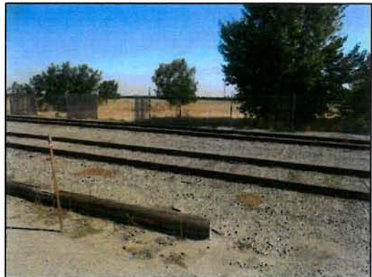
View of the east take area showing the impact on the rail spur tracks.
