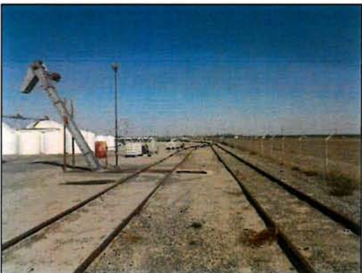
View of the rail spur that splits into two sidings.
