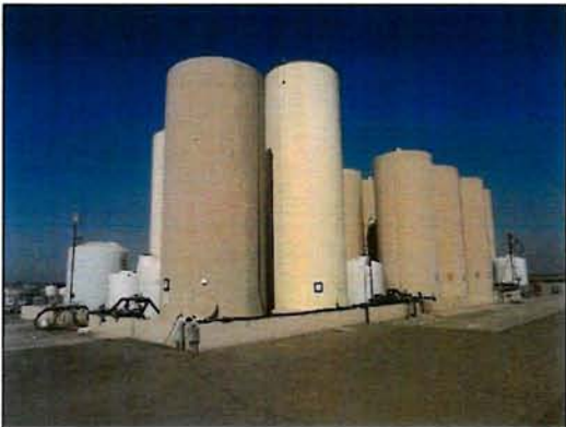
View of a tank farm with concrete containment bunker surrounding it.
