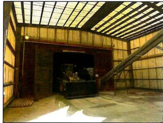
Interior view of the fertilizer storage domes.
