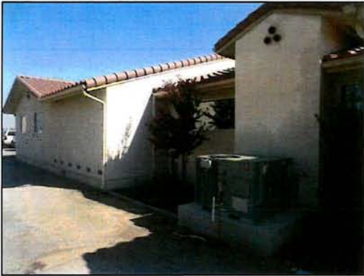
View of the west take area showing its impact on the office building.
