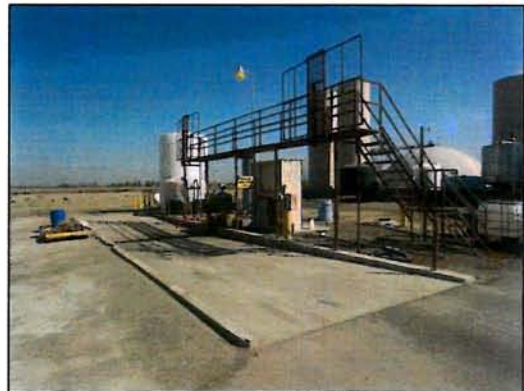
View of a product mixing station with vehicle wash rack.
