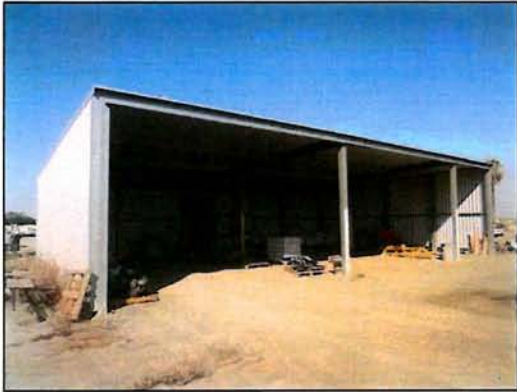
View of the equipment shelter building.
