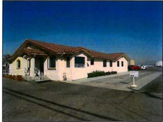
View of the office building and adjacent truck scale.
