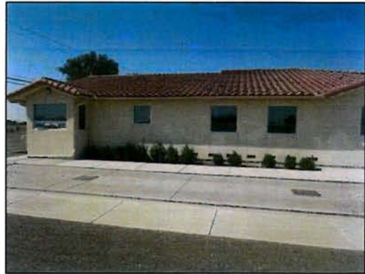
View of the west take area showing the impact on the office building and truck scale.
