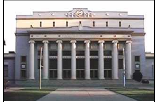
Hanford Civic Auditorium
