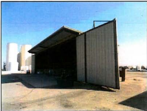
View of the product storage shelter.
