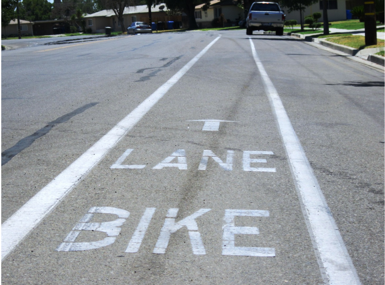
View looking south on Rodgers Road south of Grangeville Road.
