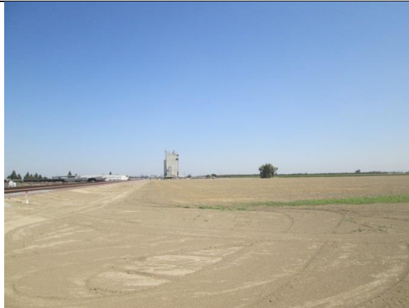
North view of rail road
