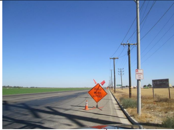
North view on 11 th Avenue
