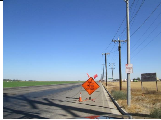
North view on 11 th Avenue
